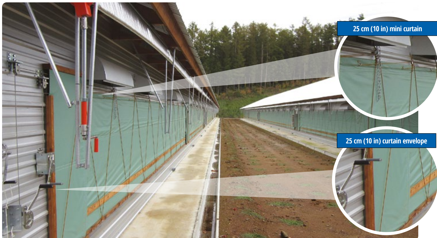
Figure 6. An example of correct curtain installation on an open-sided house.
